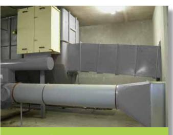
Explosion vent and outlet duct
