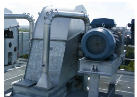
Elevators with discharge suction intakes
